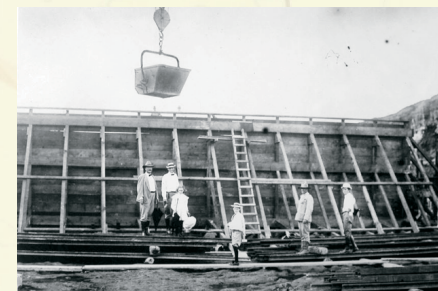
Lowering the first bucket of concrete used in the construction of the canal locks, 1908. National Archives photo no. 185-G-1893.
